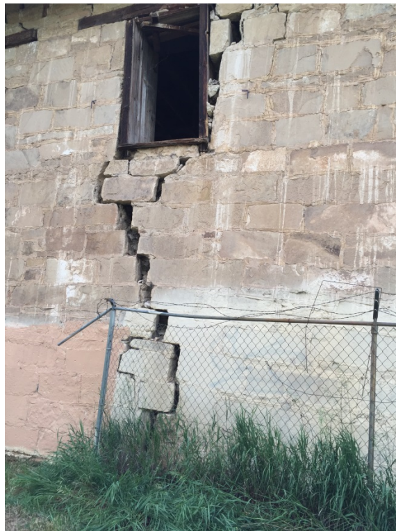
Crack on the east side of the mill.
