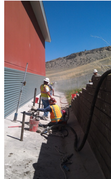
Grout Pipe Placement
