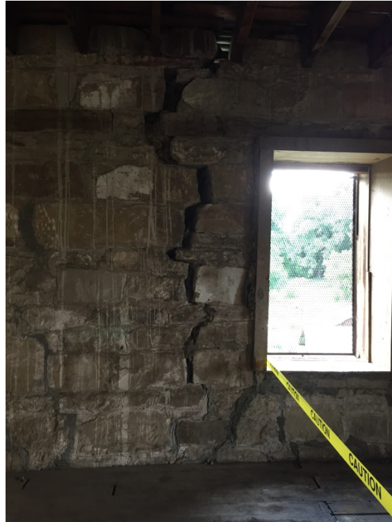
Second floor of the mill looking at the west wall crack.
